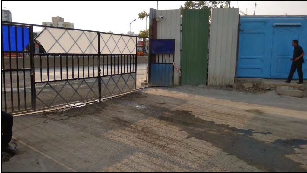
Entrance Gate area concrete done to avoid any slushy material on Road.
