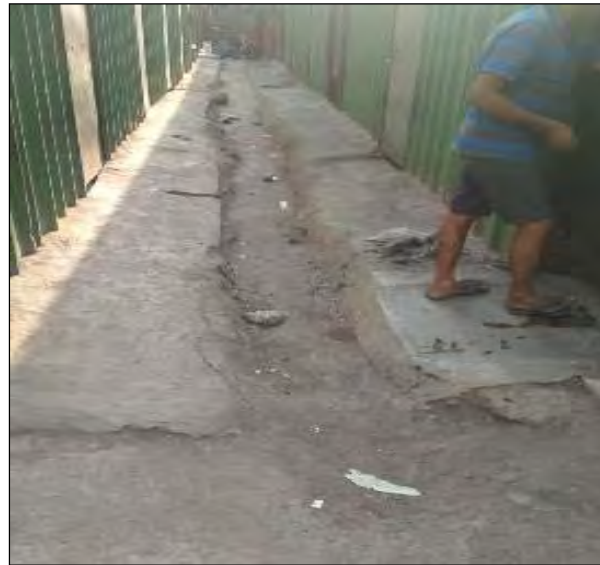
Proper Drain and slopes at labour Colony to avoid water logging
